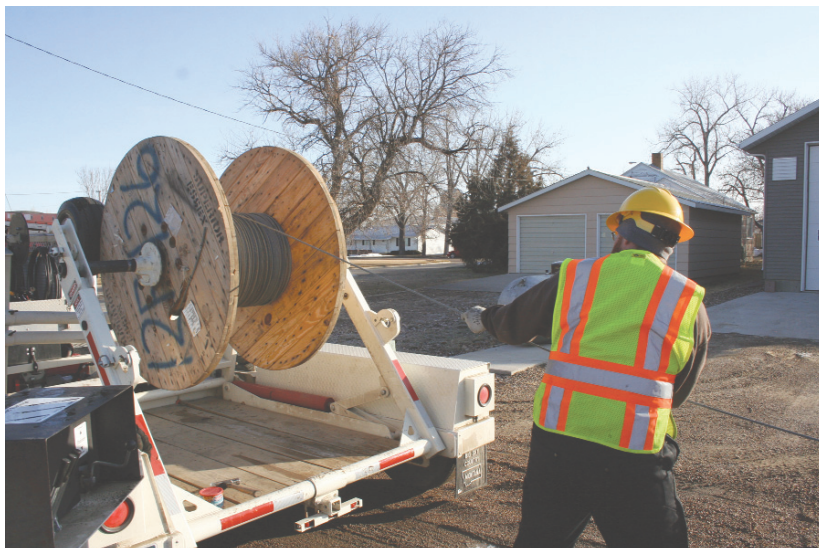
Nemont employees work hard to install fiber in upgraded exchanges
